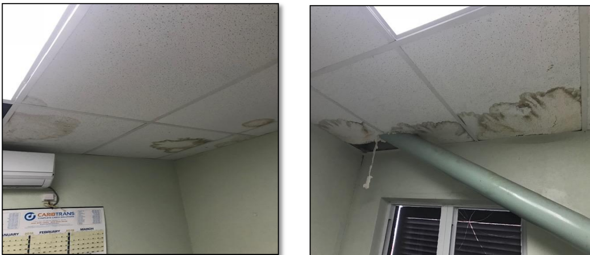
Figures K & L - Evidence of water seepage and damage to office roof
