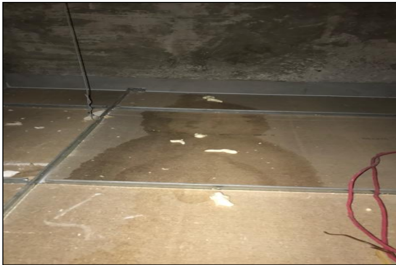
Figures E, D, F, & G - Evidence of water seepage and suspected areas of leakage in the main roof
