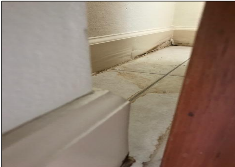
Figures A & B - Evidence of water seepage at the baseboards in MCD workspace
