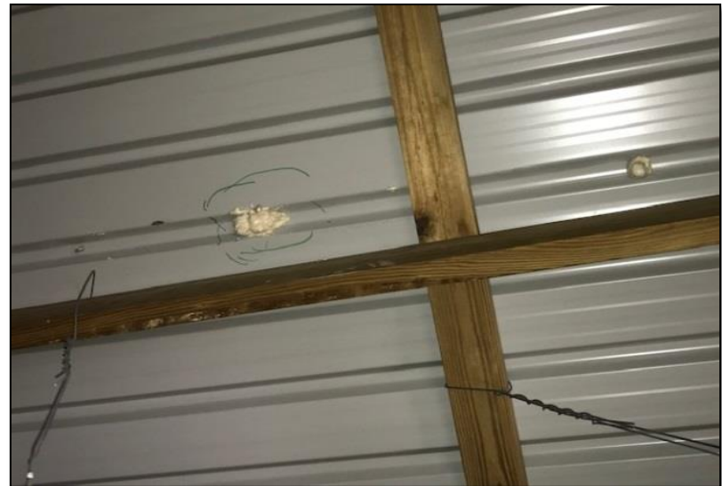
Figures E, D, F, & G - Evidence of water seepage and suspected areas of leakage in the main roof
