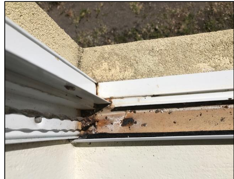
Figures C & D - Defective windows and signs of water damage
