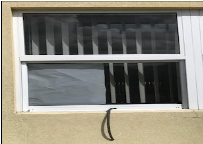
Figures C & D - Defective windows and signs of water damage
