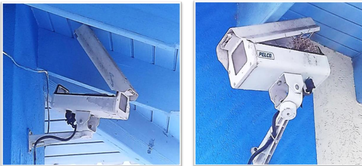
Figure L - Non-operational External Security Cameras
