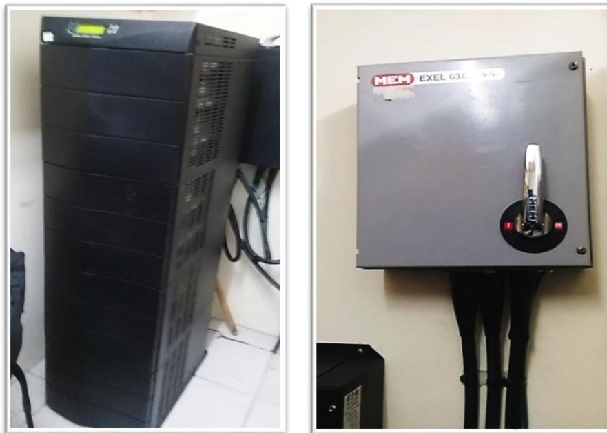
Figures D & E - RMPS Server Room 12-battery UPS Tower and Circuit Box with Metallic Emergency Safety Switch
