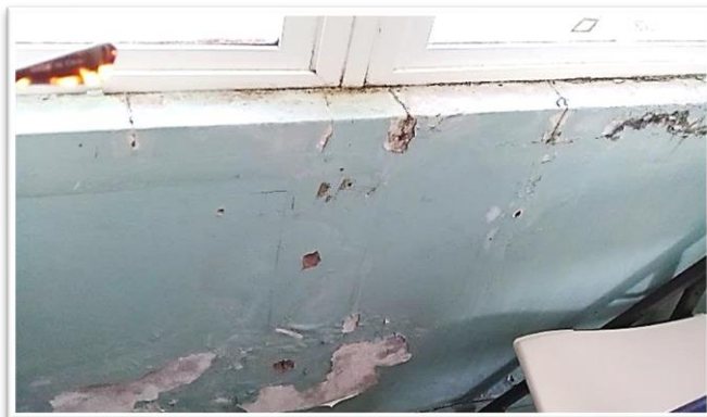
Figures XVIII & XXI - Evidence of water seepage in the Supreme Court Building
